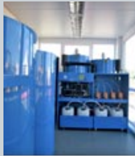
Two-stage wastewater treatment system
