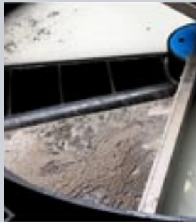
Separation of the flocculate sludge using VernEx P and aeration
