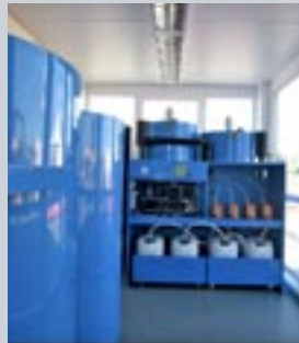
Two-stage wastewater treatment system
